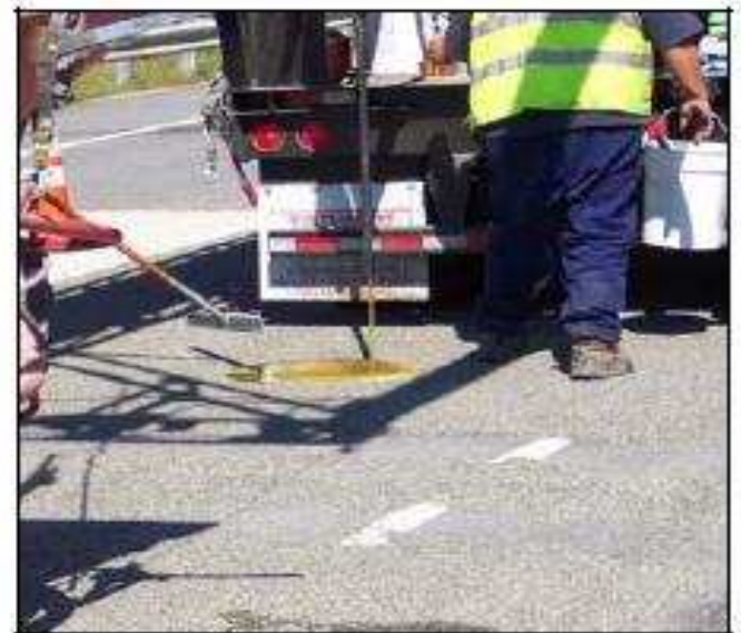
Beginning the epoxy "pour."
