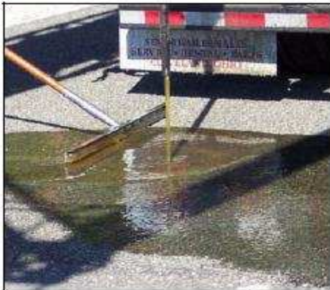
Crew uses squeegee and roller to distribute product across deck.
