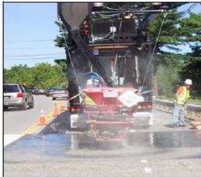
Aggregate is carried from hopper by conveyor and distributed over the epoxy.
