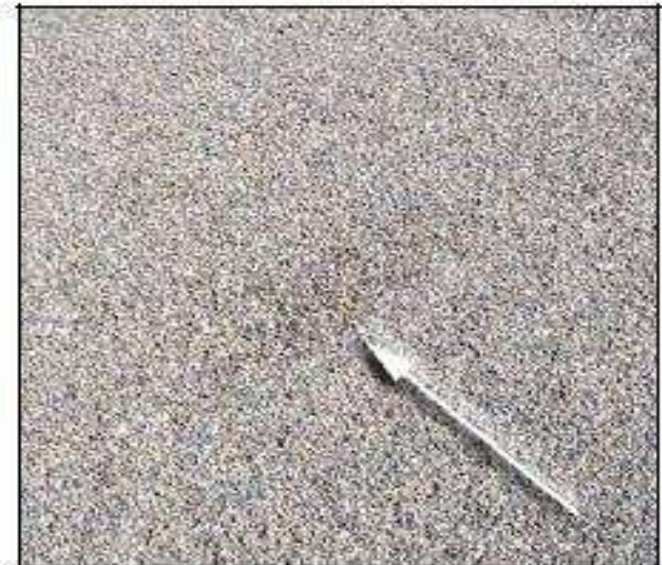
Material is disbursed by hand to areas where epoxy comes through.
